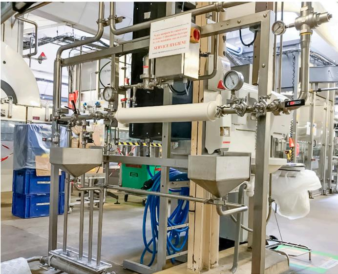
Figure 7: Capsule Filter Horizontal Installation at POU
