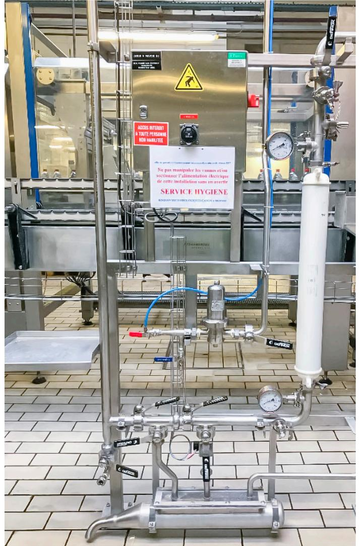
Figure 8: Capsule Filter Vertical Installation at POU
